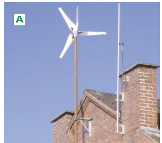
Ampair 600 on brick wall mount
