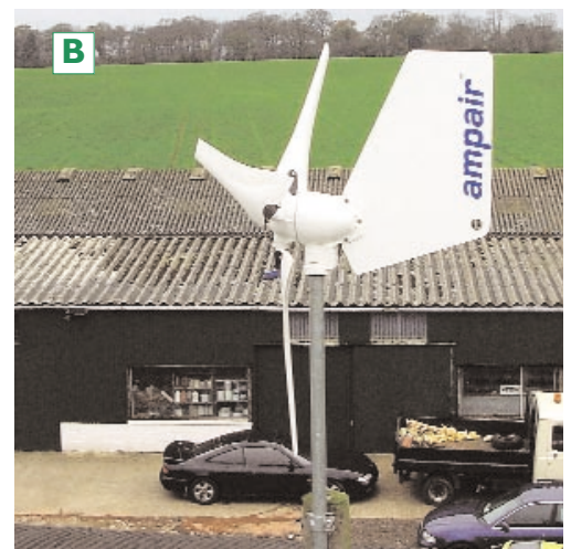
Ampair 600 on telegraph pole mount
